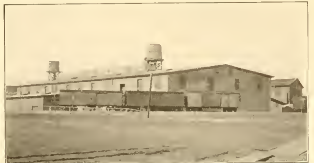
PART OF PRESENT PLANT, WEST END.
